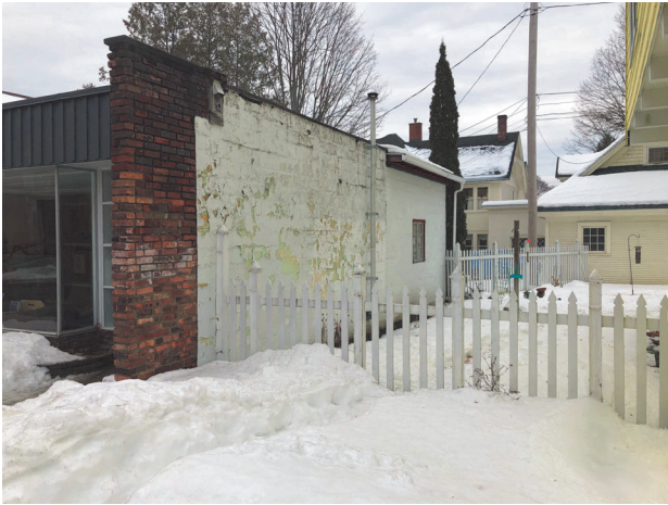
4 View of Existing West Wall
