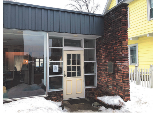
3 View of Existing Entry
