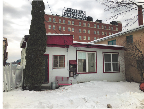
5 View of Existing South Wall
