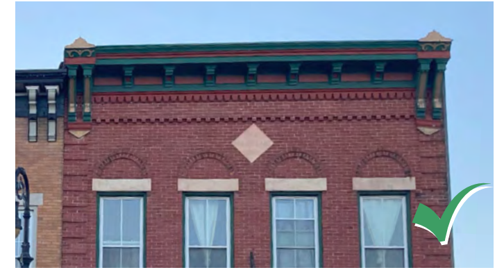
Restore and paint original pressed metal cornices to highlight detailing.
