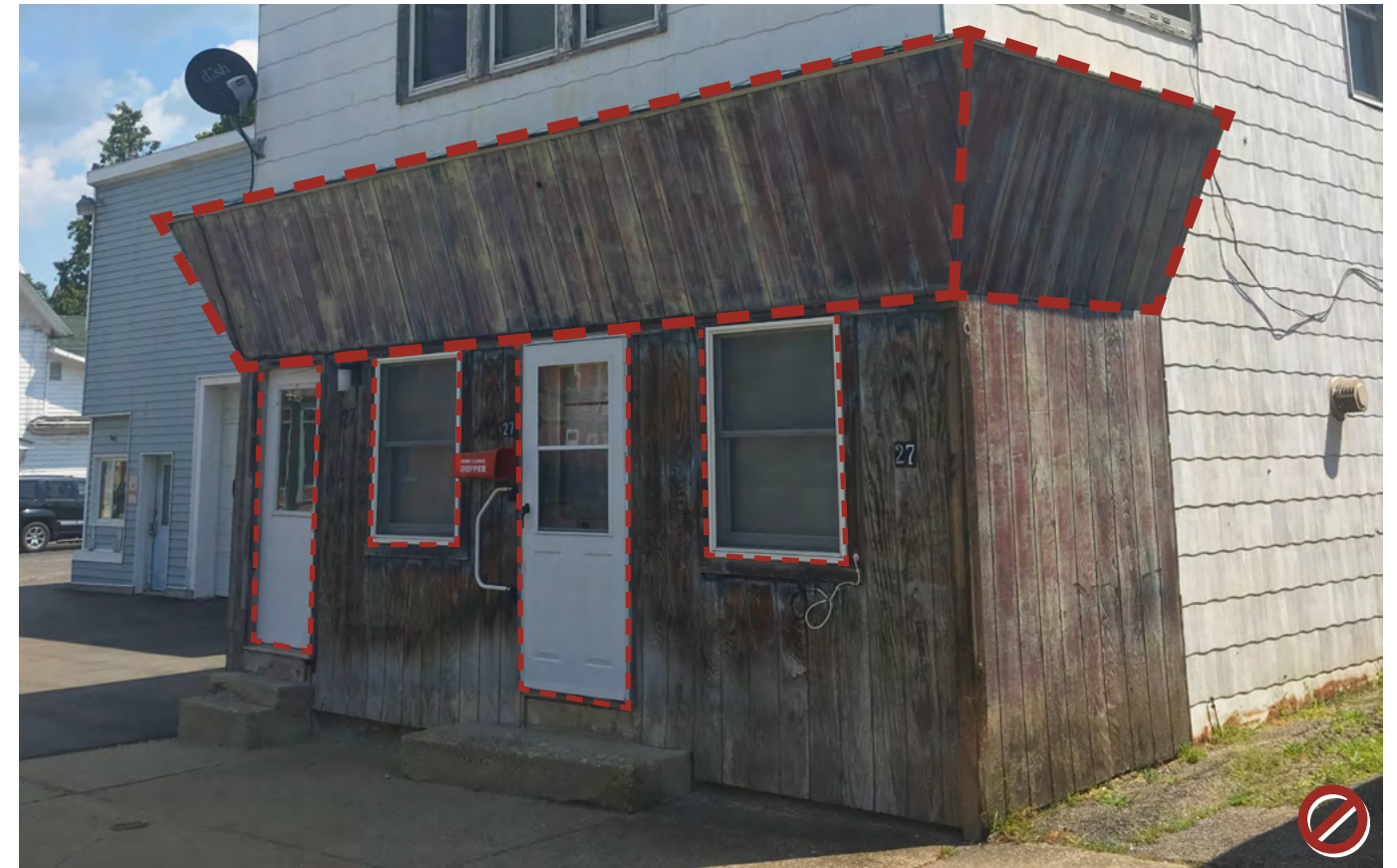
Do not cover up original cornices or transom windows with structured awnings or oversized signage areas. Do not place residential vinyl windows and doors on commercial storefronts.
