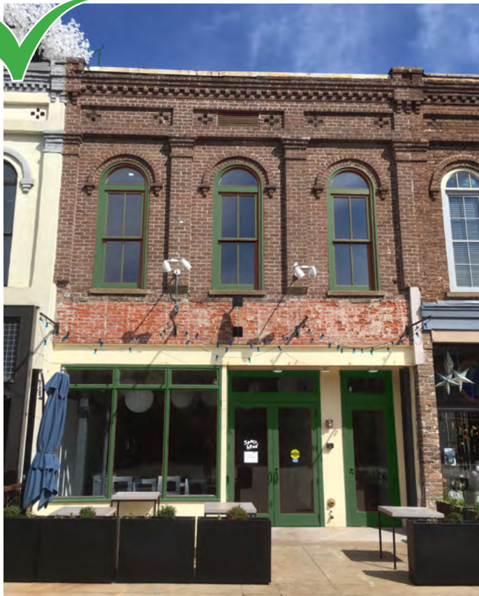
Color can be applied to new window and door finishes to breathe new life into a historic facade.
