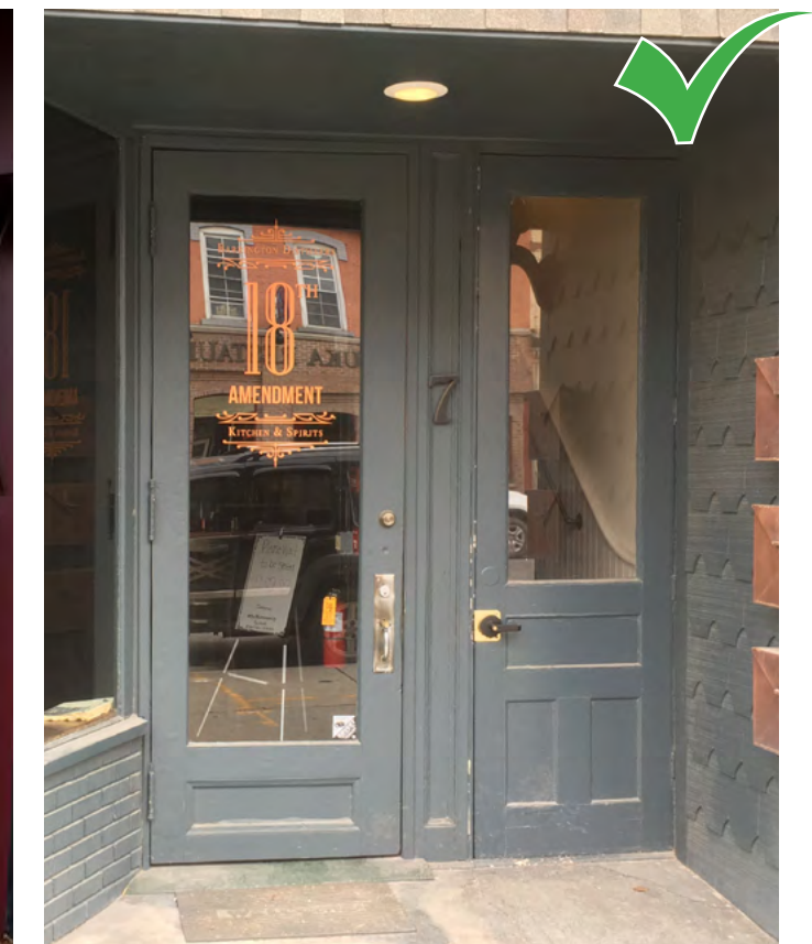
Do use full glass entry doors for storefronts and half glass doors for residential upper floors.
