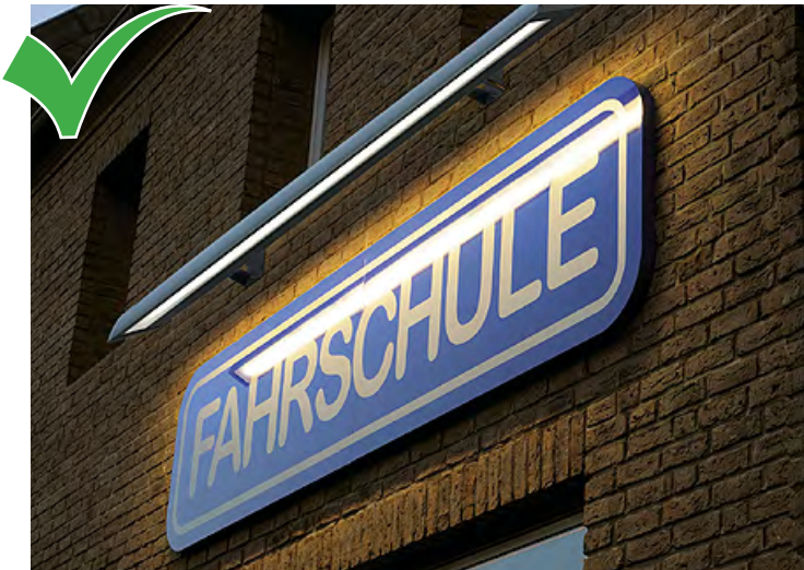
Use linear light fixtures for wall signs and other horizontal surfaces that need even lighting.
