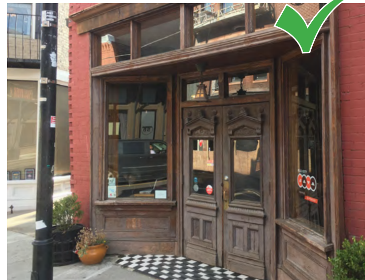
Historic wood windows can have a long lifespan if properly maintained.
