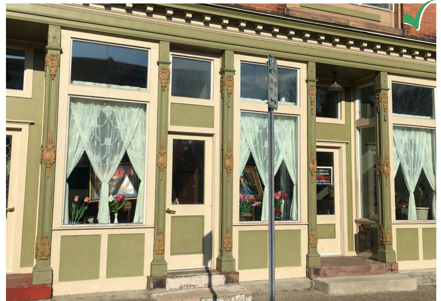
Use materials that can be repaired and maintained similarly to the original - such as fiber cement in place of wood.
