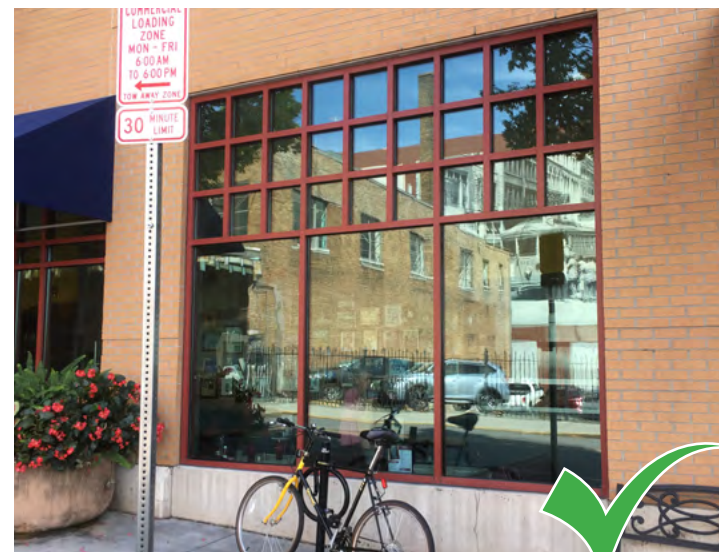
Use a variety of window sizes and patterns on new windows to reduce scale.
