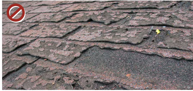
Replace asphalt shingles that are past their lifespan with a more durable alternative.
