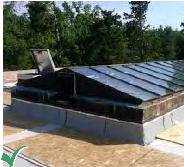
When possible, restore or repair original rooftop features such as skylights.
