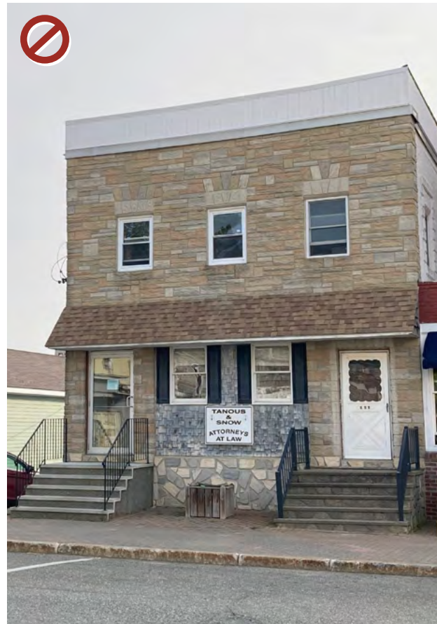
Siding replacement should match the materiality of the original building. Wood with wood. Masonry with masonry.
