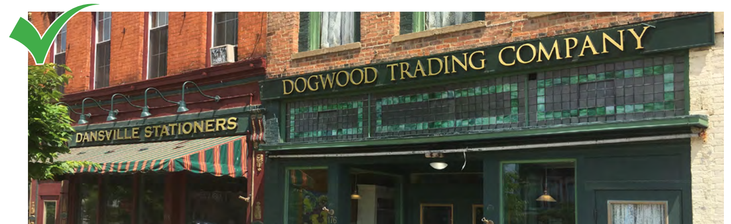
Wall signage should be legible, but not overshadow the architectural character of the facade.
