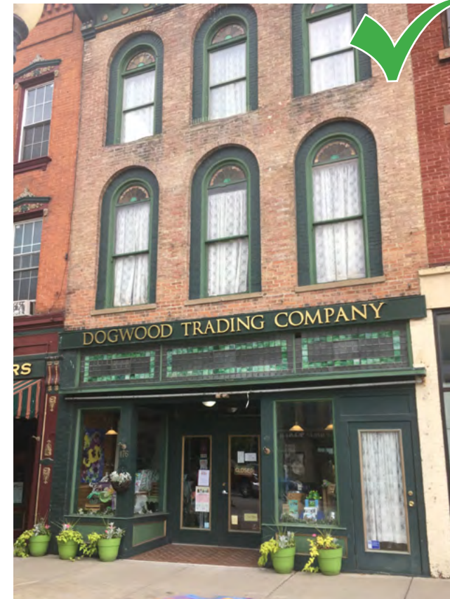
Match color schemes with original materials - such as stained glass transom windows.
