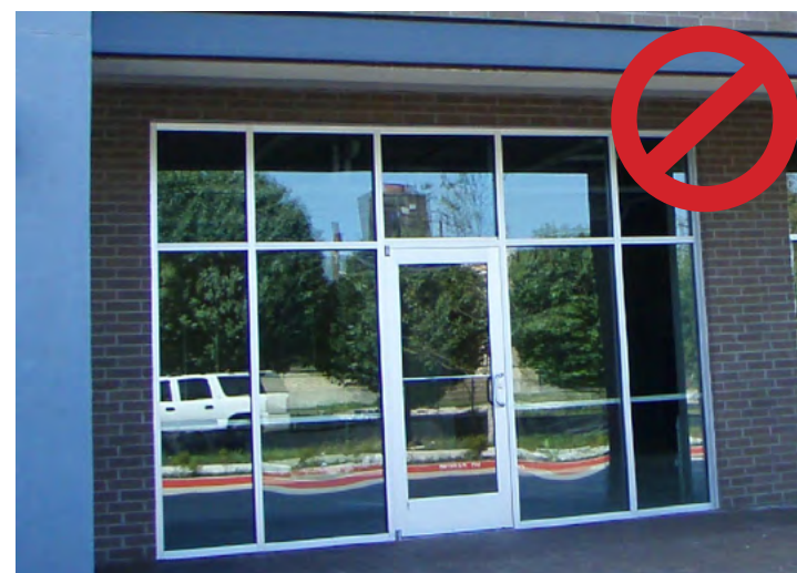
Do not use floor to ceiling tinted glass or prefabricated metal storefronts
