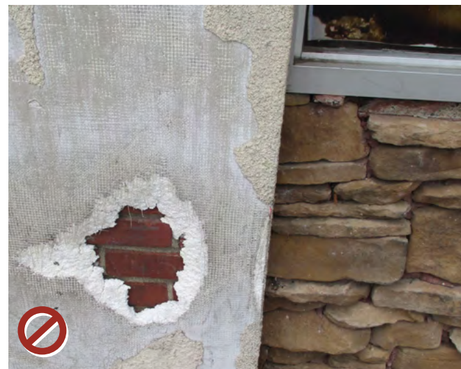
Do not use EIFS to cover original materials or in places requiring durability.
