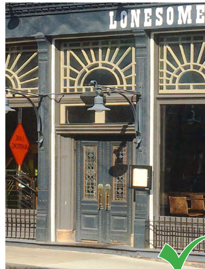
Restore historic detailing on and around doors and openings. Use color to highlight detail.
