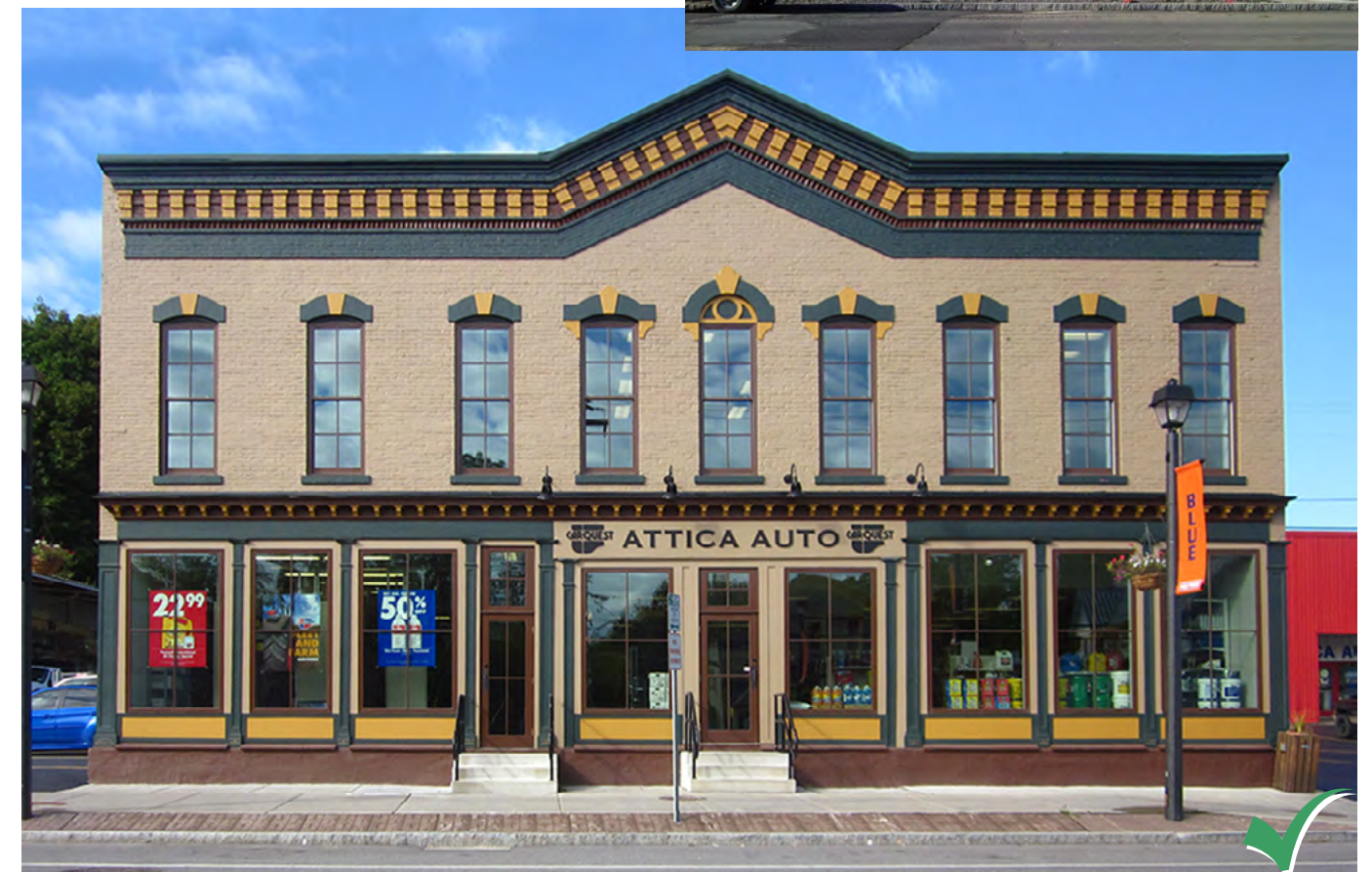
Restore original window openings that have been covered up over time. Highlight original masonry details with contrasting paint color schemes.
